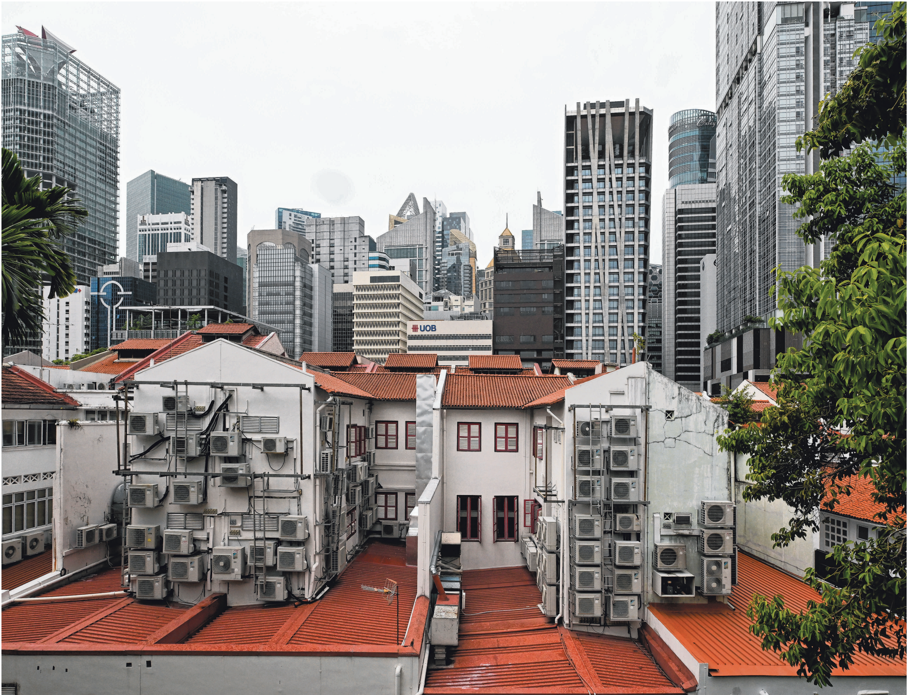
Air-conditioning units at the back of shophouses in Amoy Street in 2022. Air-conditioning has become an integral part of the daily lives of Singaporeans, be it at home, in the office or at the shopping mall, says the writer. But this love affair comes at a cost – both economic and environmental. ST PHOTO: LIM YAOHUI
